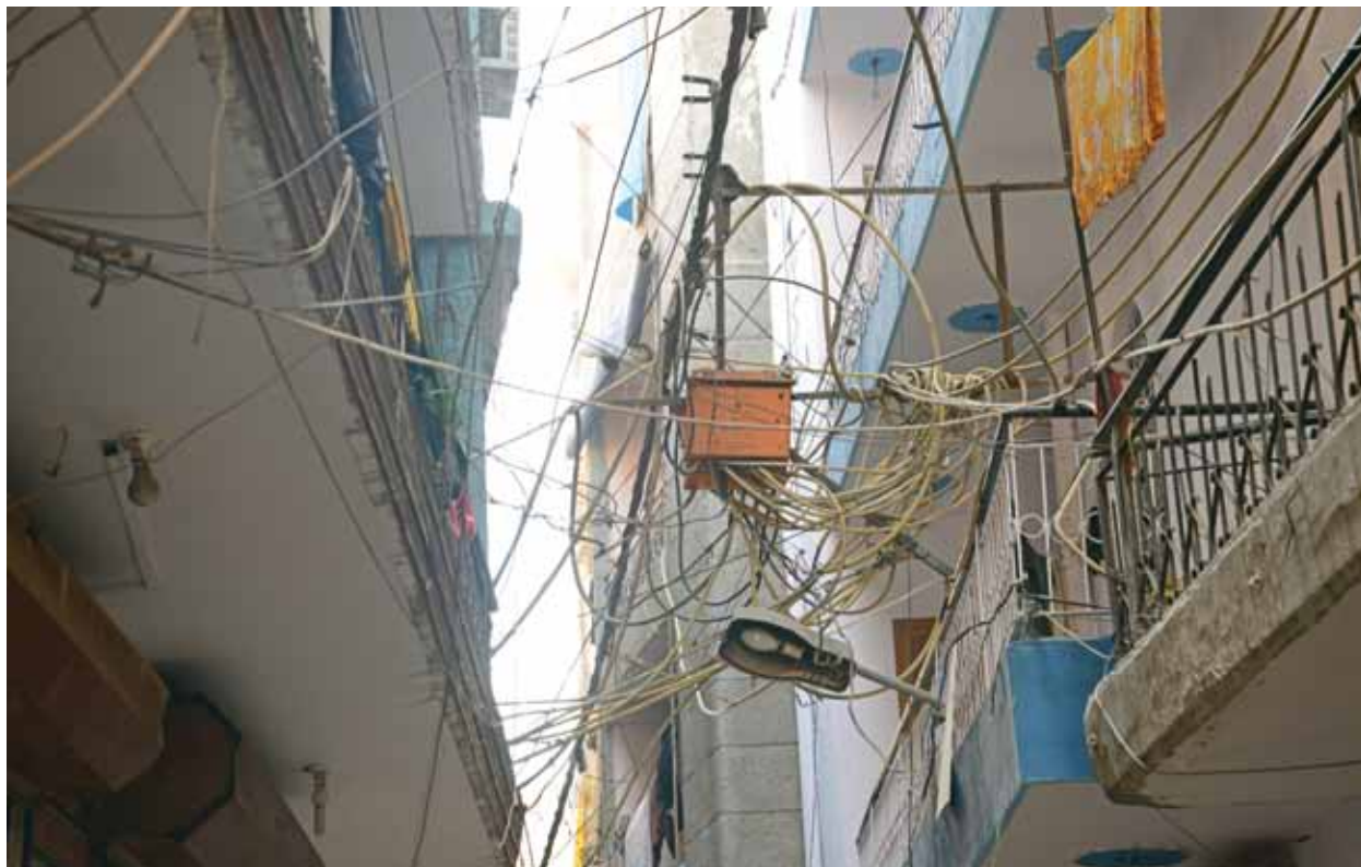
The electric poles and the maze of electrical wires need to be urgently removed and new technologies should be adopted keeping in mind safety and aesthetics.
