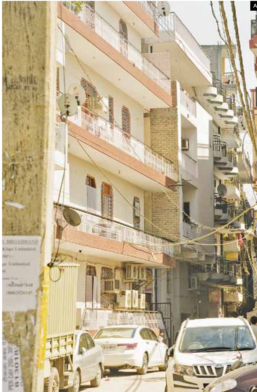
The newly-built houses have very good construction and are being rented out to IT companies.
