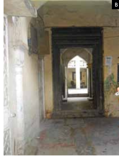
The gully from street to courtyard in some old houses
