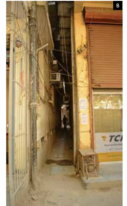
The gap between two buildings is too narrow and unsafe
